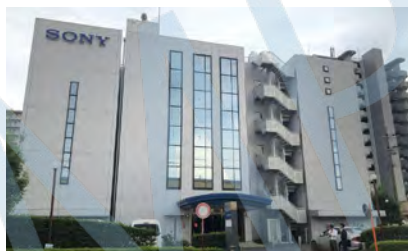
SFI Omiya Building (Omiya, Saitama City) No. 10 in Table (B) Rio Consulting (S) Sony (T) Unicharm, Sony Marketing
