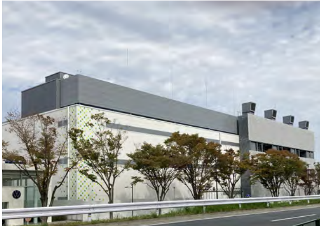
TKW1-1 under construction in Tama City, Tokyo, by GLP. Photographed in October 2024.
