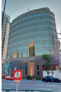
Former Goldwin Headquarters Building (Shoto, Shibuya-ku) No. 2 in Table ⓑ First-Corporation Ⓢ Raysum
