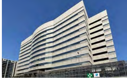
Canal Side Building (Shinagawa, Shinagawa-ku) No. 3 in Table ⓑ Haseko Corporation Ⓢ Open House Development
