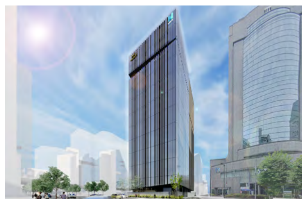
Rendering of Kobunacho Project to be developed by Hulic. Prepared by Nikken Sekkei, which is engaged in the design. (Courtesy of Hulic)
